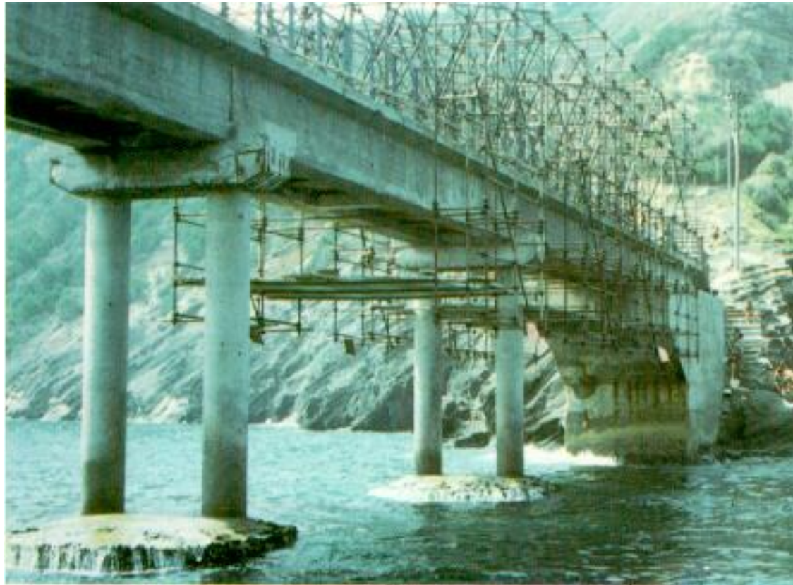
CASSONETTO BRIDGE - ITALY
