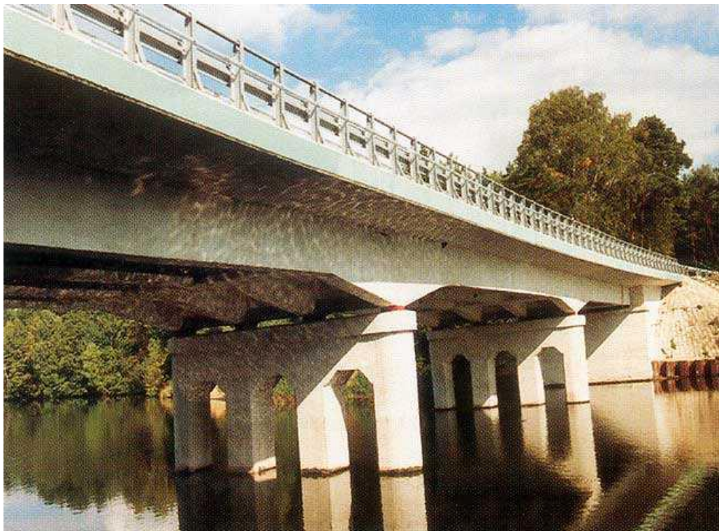
KRYNICA BRIDGE (POLAND)
