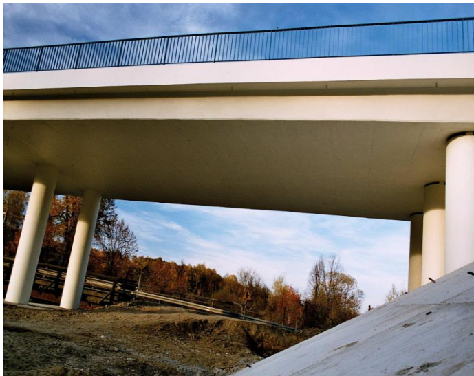
BRIDGE IN BYDGOSZCZ (POLAND)
