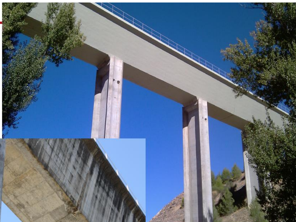
AQUEDUCT IN ZAFRA (SPAIN)
